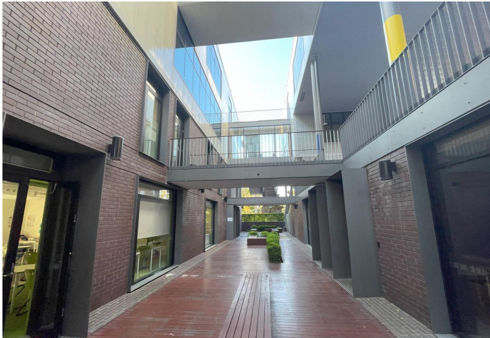
Figure 4. Building A, level 0 classrooms
