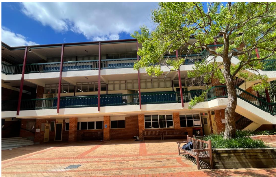
Figure 7. View of northern elevation, Building J (Level 2 - Science Labs)
