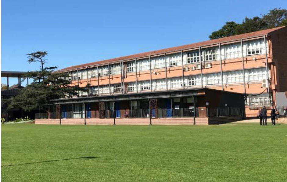
Figure 4. Northern elevation of Building H with demountable building in the foreground
