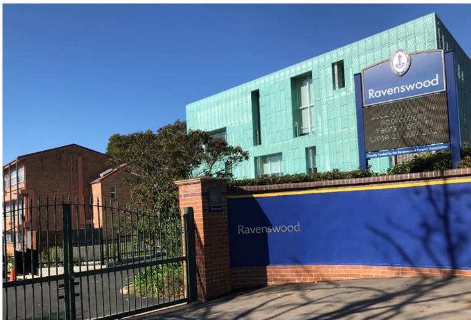
Figure 8. View of recently constructed SLC from Pacific Highway entrance
