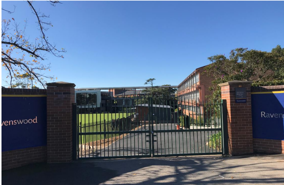
Figure 7. View of the demountable building (centre) through school gate at the Pacific Highway entrance
