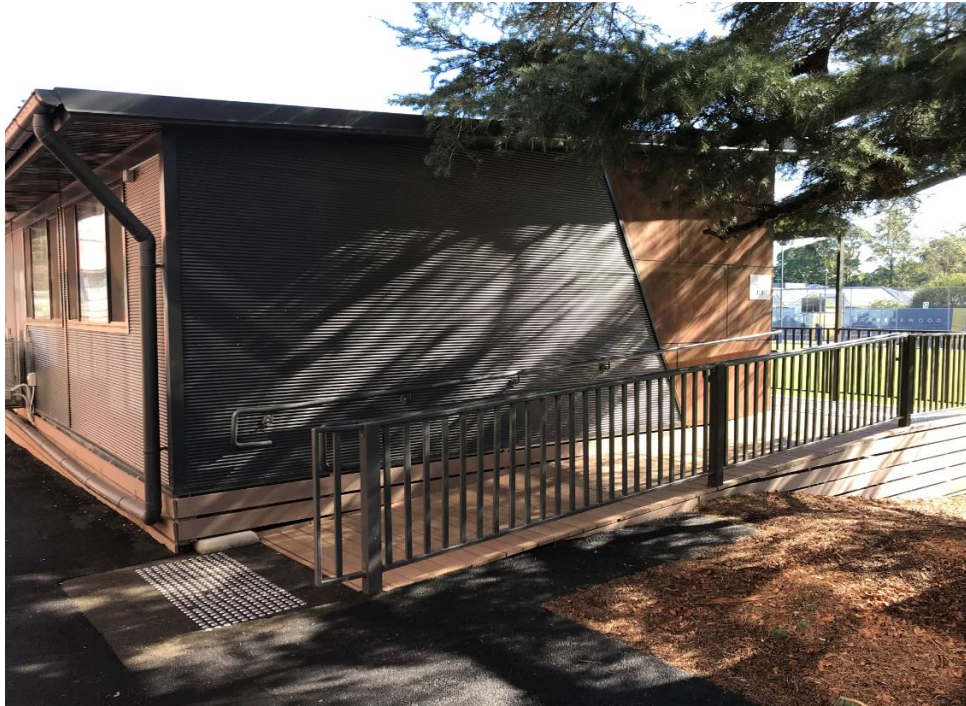
Figure 5. Eastern elevation of the demountable building
