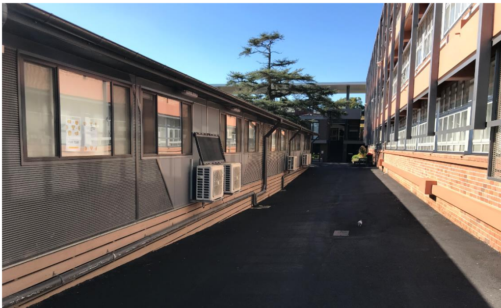
Figure 4. The southern elevation of the demountable building (to the left)
