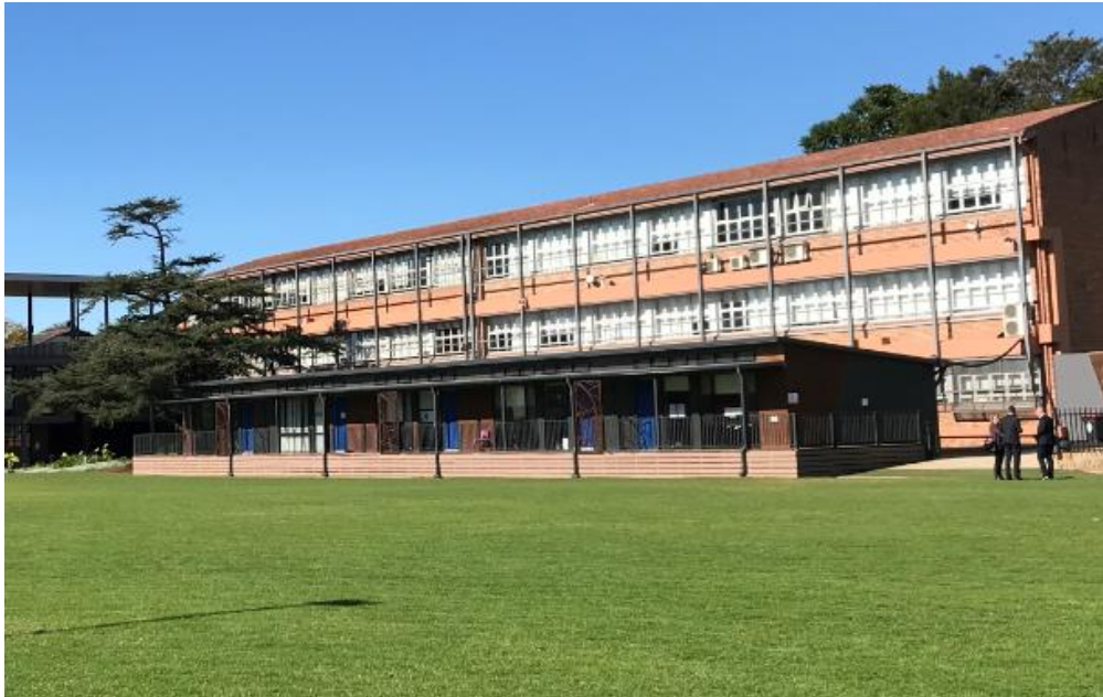
Figure 3. Northern elevation of the demountable building (in foreground)
